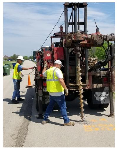
on the streets, these were locations of bore holes for the geotechnical analysis. Contractors were out in the village last week taking samples of the existing road surfaces and the ground under our roads. Our engineers will use the results of the analysis to develop a preliminary road profile design. I have asked Kimley-Horn to present the Geotech results and their preliminary designs at our May meeting.
