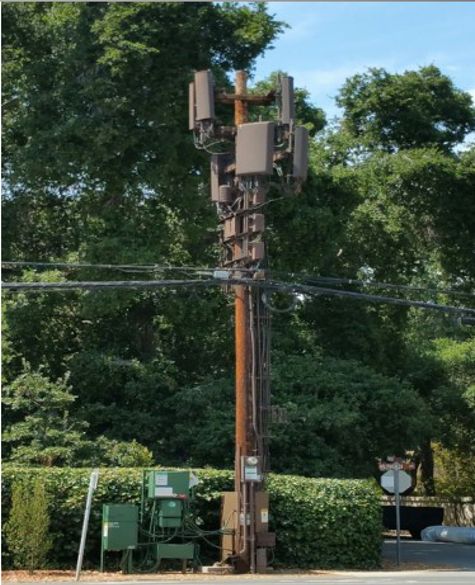
Example of a cluttered small cell install
